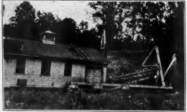
View of Dredge and Jet
